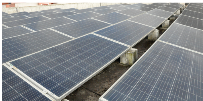
One of the 'Best Practices' of the college- Installation of 120kWp Solar Grid Roof Top PV System to generate Non-conventional renewable energy.
