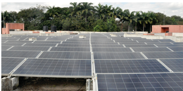
One of the 'Best Practices' of the college- Installation of 120kWp Solar Grid Roof Top PV System to generate Non-conventional renewable energy.
